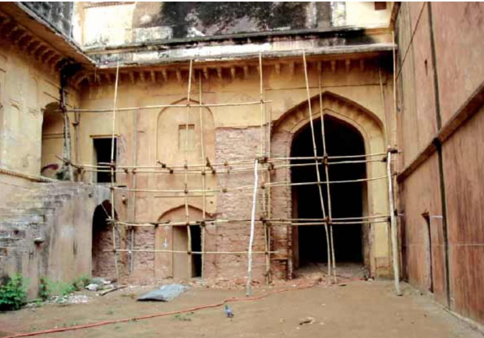
West court area, passage being repaired
